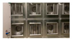
An integral component of the upgrade to the Renown Health Institute for Cancer Radiation Therapy was the installation of a fan wall with Automated Logic controls to help remove airborne contaminants and improve IAQ.
