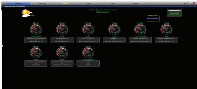
Real-time pressure differential monitoring across FreeFlex production zones replaces manual logging.
