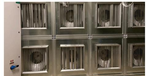
An integral component of the upgrade to the Renown Health Institute for Cancer Radiation Therapy was the installation of a fan wall with Automated Logic controls to help remove airborne contaminants and improve IAQ.
